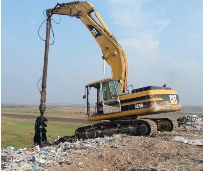
Drilling of degas wells, Arad, 2014.
